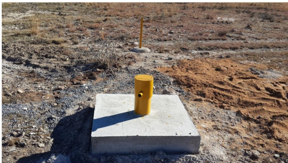
Figure 31: SD1-16 Completed Headwork's
