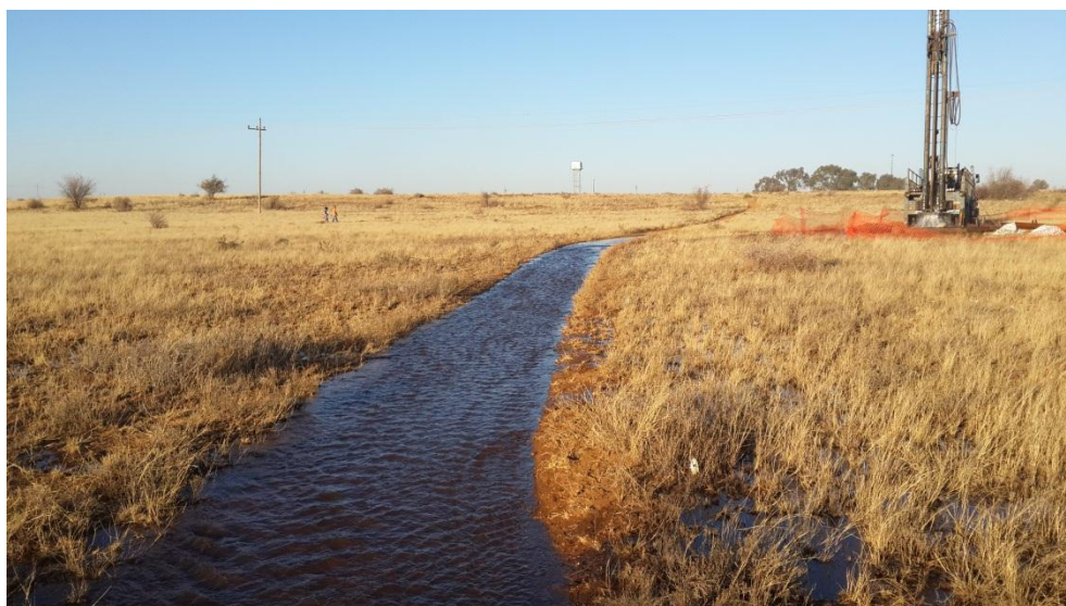
Figure 33: Drilling of SD1-45 Danielskuil Municipality Supply Borehole
