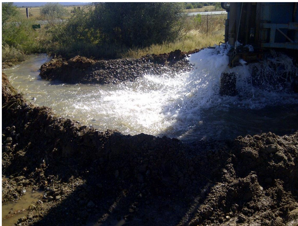
Figure 26: Drilling of SD1-08 - BY 38.9l/s
