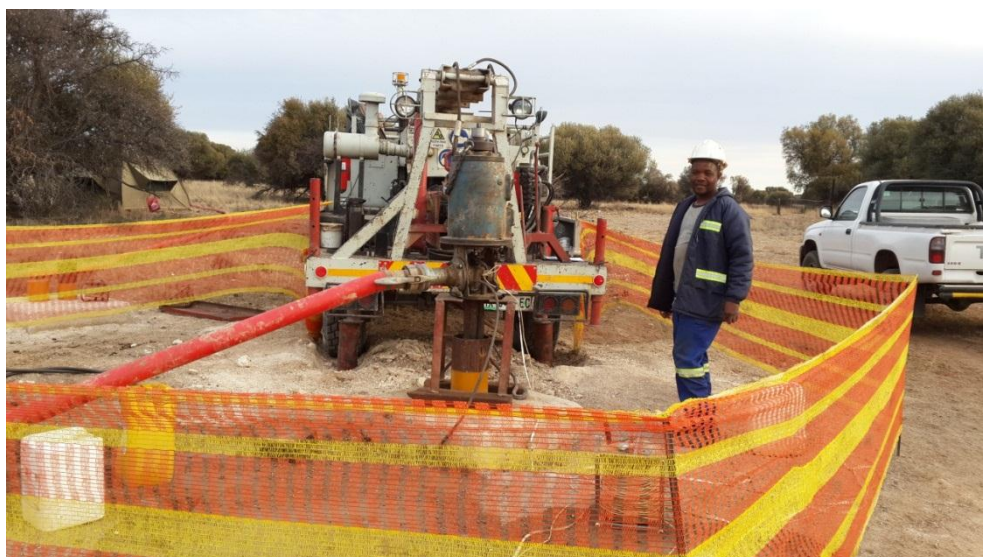
Figure 37: Aquifer Testing SD1-27
